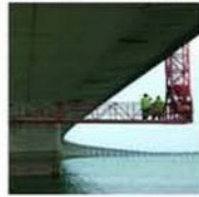
Structural Maintenance Engineering
