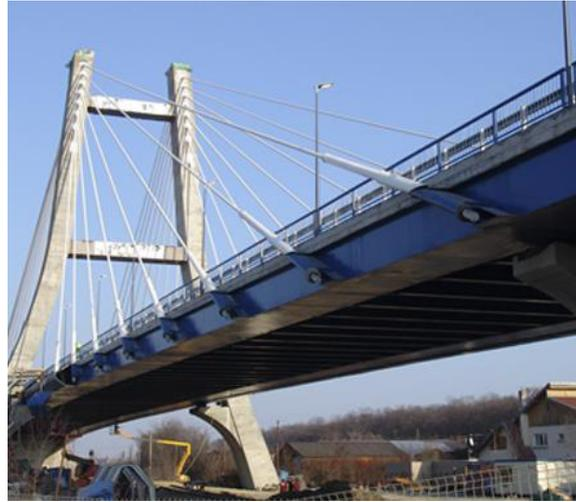
The "Centura Bridge" has a 35+85+85+35m span distribution, with a central pylon and two intermediate piers. The need of these piers rises from the impossibility of building a taller pylon due to height restrictions imposed by the proximity of a nearby airport.
